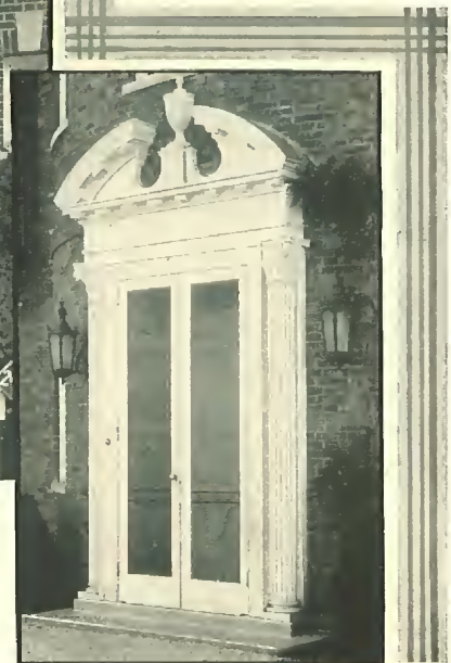
Here (right) is a pair of single panel doors perfectly designed and proportioned. These doors have two bronze rods let into the door stiles serving as braces for added rigidity and as push bars.
